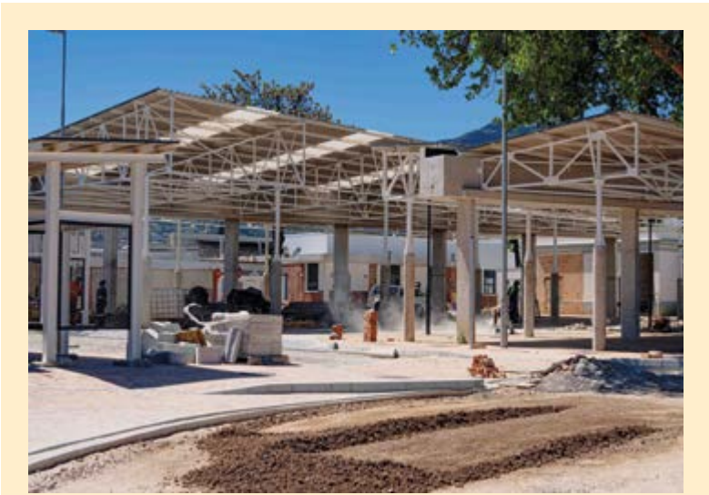
CFM, your PTI is coming! Construction of the public transport interchange (PTI) in Somerset West is on schedule and will be complete by May 2024. The PTI is located on the corner of Andries Pretorius and Victoria streets and will serve an estimated 1 000 commuters and 300 minibus taxis every weekday. Destinations served will include Lwandle, Macassar, Firgrove, Strand, Nomzamo, Sir Lowry's Pass Village, Zola, Khayelitsha, Stellenbosch, Somerset West and Grabouw.
